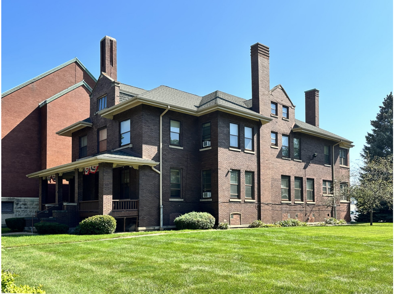
For the design of the rectory located at the western end of the complex, pictured above, the architectural detailing at the exterior is modest and restrained. Each elevation is accentuated by deviations from the main floor plan including the semi-enclosed front porch and gabled wall dormers which break through the roofline at the wide eaves of the hipped roof.
