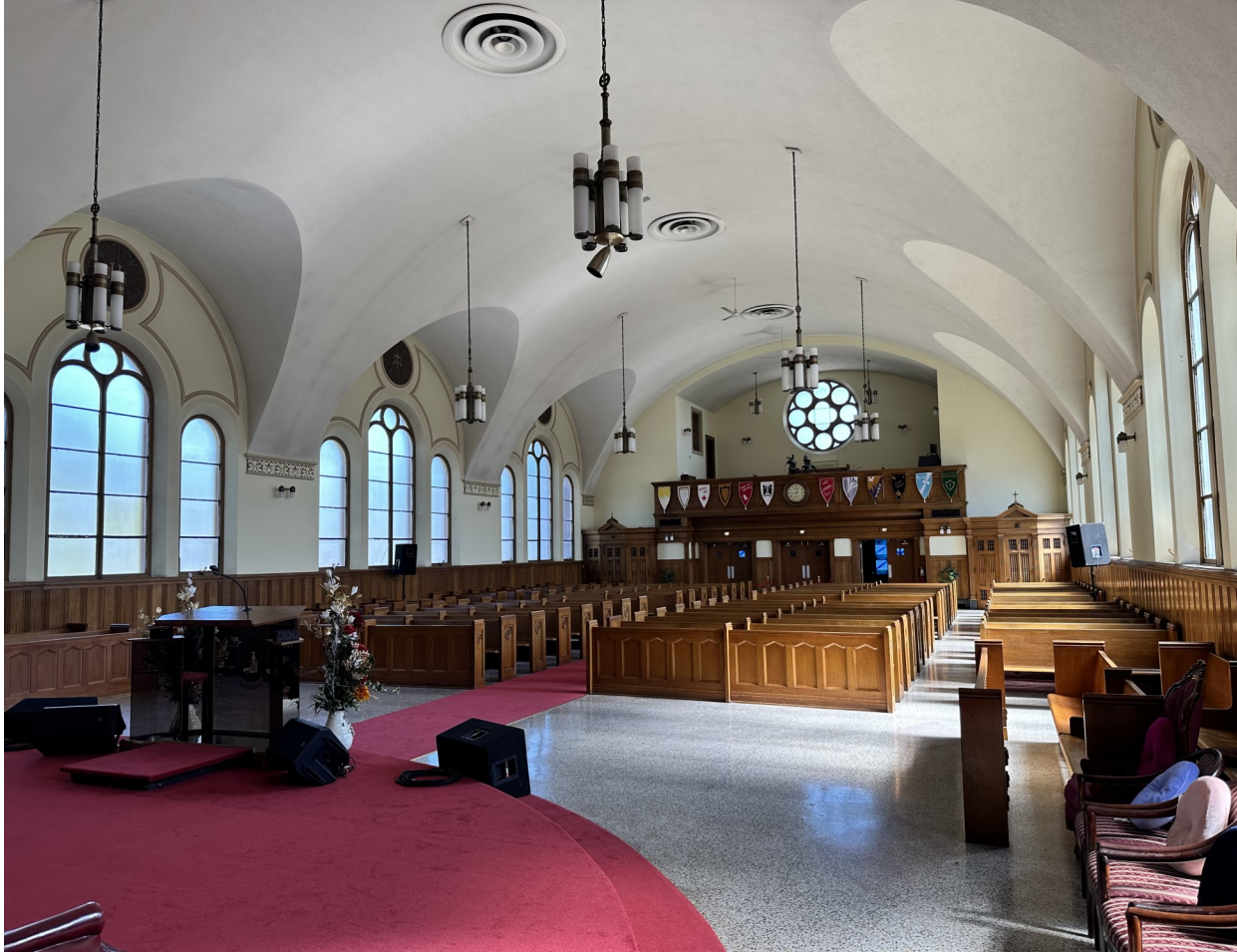
Pictured above is the sanctuary for Greater Tabernacle Cathedral which shows the soaring groin vault ceiling, monumental arched windows, and historic finishes following the 1937 fire.
