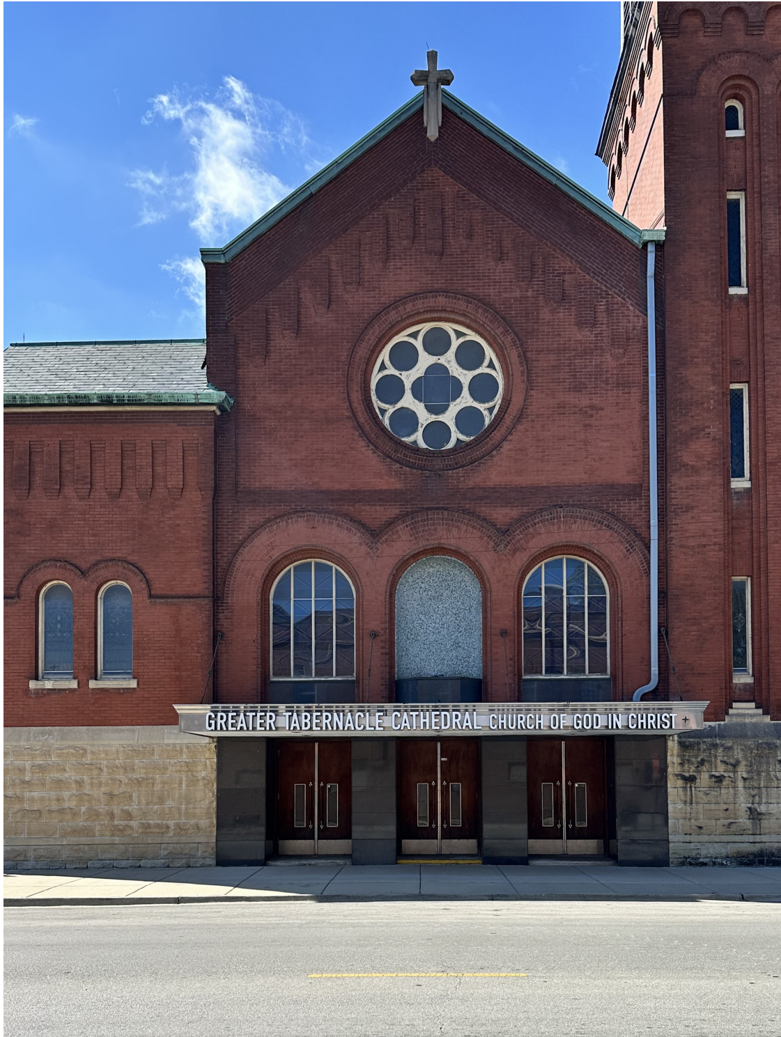
At the former Holy Rosary Church, Beman designed a magnificent and impressive exterior with a classical monumentality. Pictured here is the central bay of the east façade of the church which features a heavily rough hewn Joliet limestone base, a striking arcade trimmed in brick relief work, and a grand rose window. The bay is crowned by a prominent front facing gable adorned with brick corbeling at the face of the gable and a stone cross at the peak.
