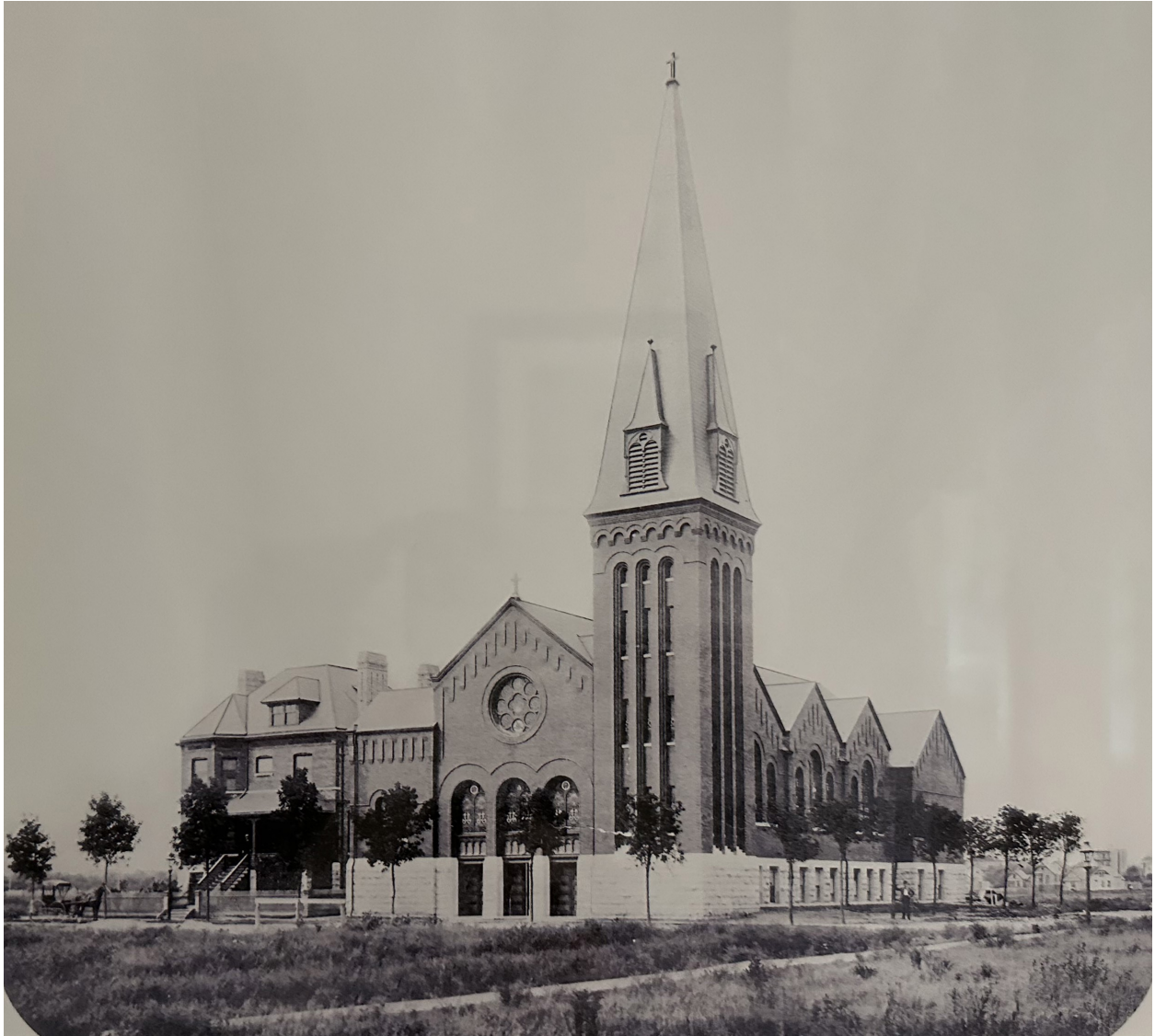
Greater Tabernacle Cathedral, formerly Holy Rosary Parish, was the first Catholic parish established to serve the Roseland-Pullman Community. Its significance as the center of Catholic life in the community is illustrated by the monumental architecture of the extant church building. When the church was first completed it was an imposing edifice on the vast rolling prairie previously dotted with Dutch farmhouses and homesteads. Pictured above is a photograph of Greater Tabernacle Cathedral shortly after its completion in 1890. (Credit: Archdiocese of Chicago Archives)
